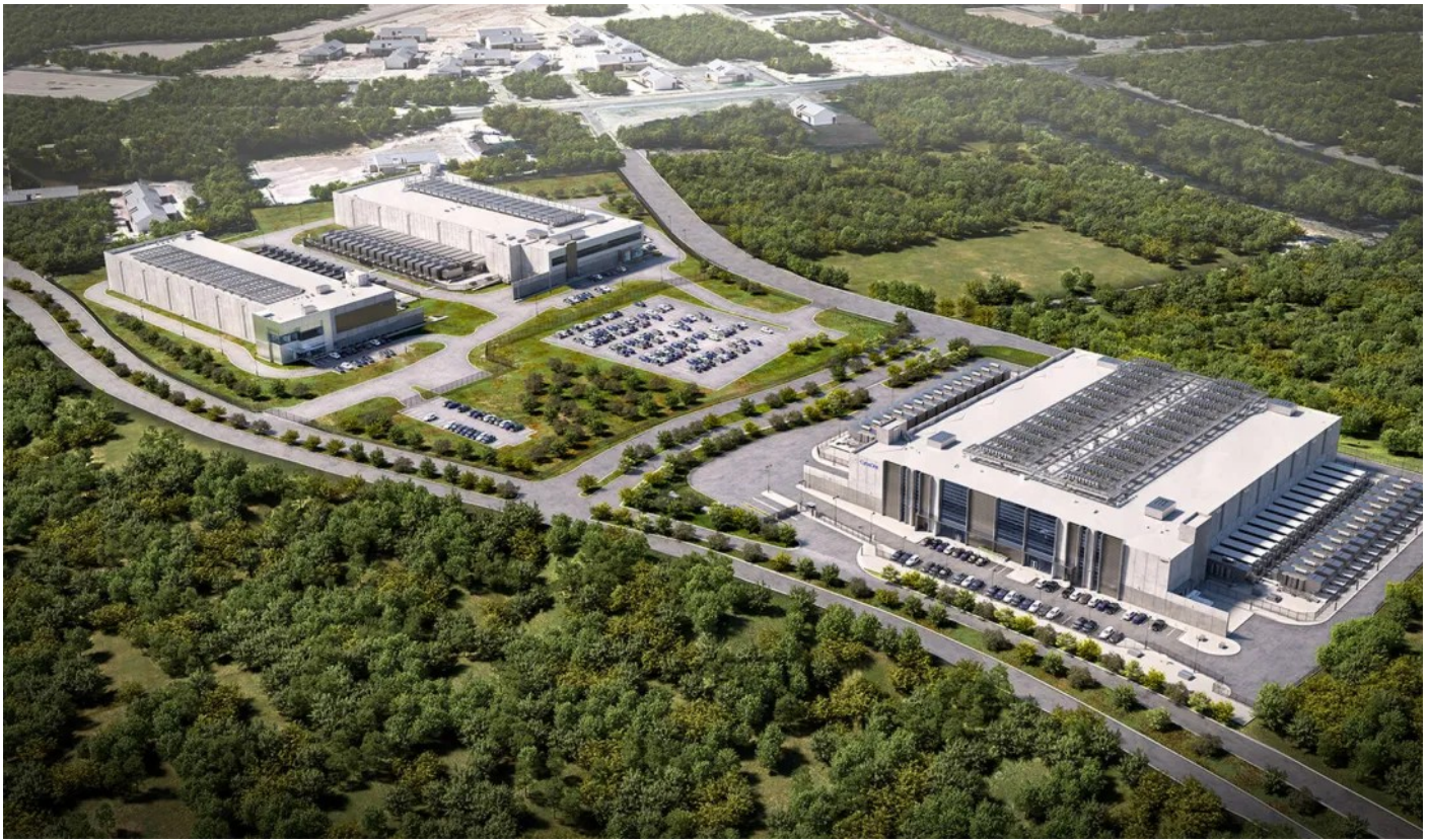
San Antonio data center campus
